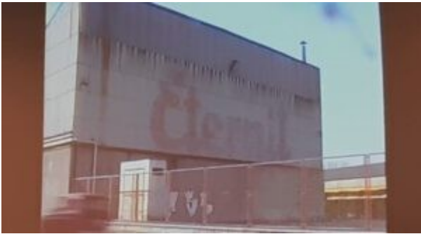
The Casale Eternit plant
